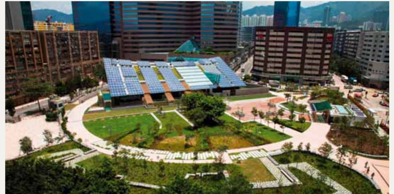
The new building in Kowloon Bay not only has zero net energy consumption, but actually feeds green energy into the grid.
