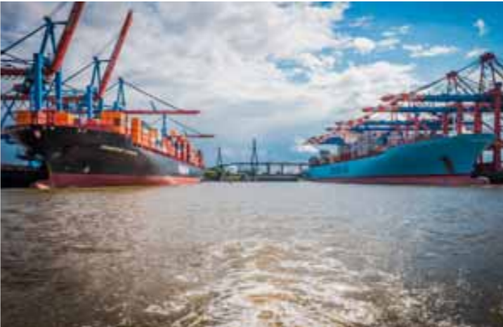
By using onshore power rather than the ships' diesel engines, port cities can massively reduce emissions.
